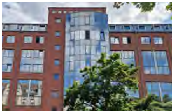
Figure 15: Exterior view of the office building in Berlin, source: FIZ Karlsruhe, Franziska Fodstad
